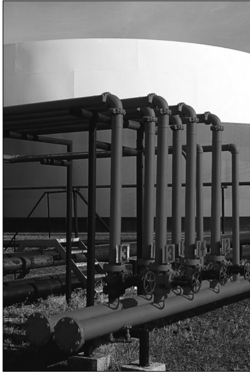
Steam pipe bridge in a geothermal power plant. Pipe flows are everywhere, often occurring in groups or networks. They are designed using the principles outlined in this chapter. (Courtesy of Dr. E. R. Degginger/Color-Pic Inc.)
